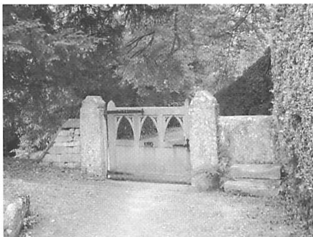
Bibury - Bibury churchyard with an unusual dry stone wall roofed with Cotswold stone tiles.
