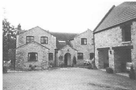
Pete's beautifully restored house in West Staughton
