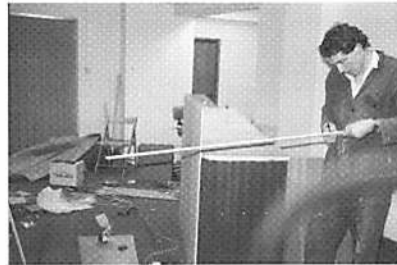
20-5-85, 9.45 pm. The ‘chippy’ constructing the reception desk
