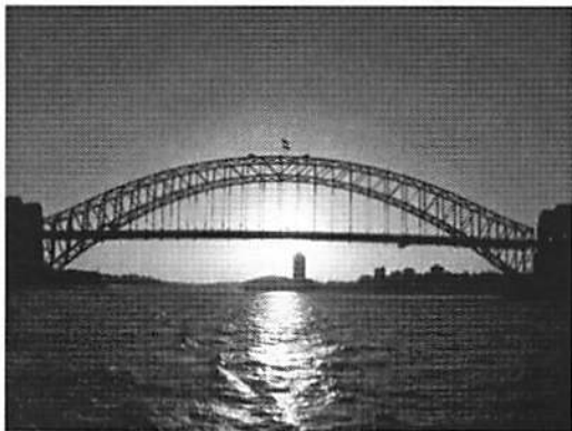
Sydney Harbour Bridge
