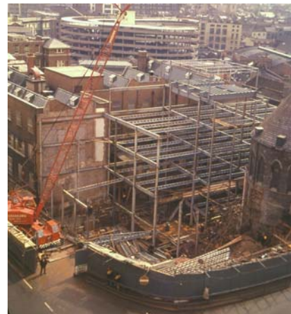
The 1964 extension under construction
